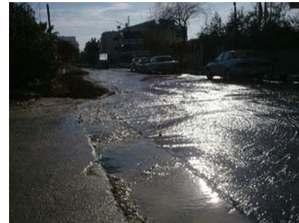
More than %50 of potable water is lost
