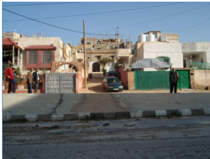
Four houses which have jointly covered the cost of a long connection to the nearest sewerage line
